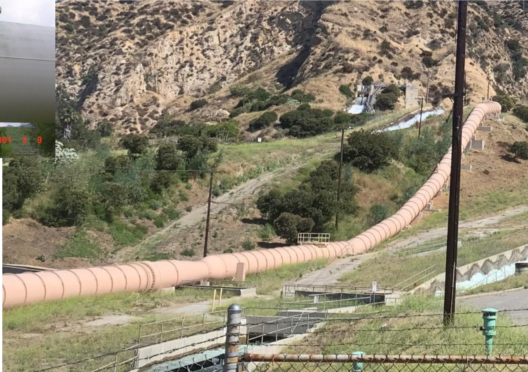
Ring girder on pile supported pier, damaged from lateral spreading 1971 & 1994
