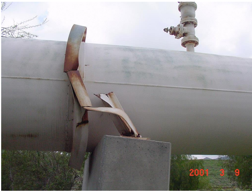
Ring girder on pile supported pier, damaged from lateral spreading 1971 & 1994
