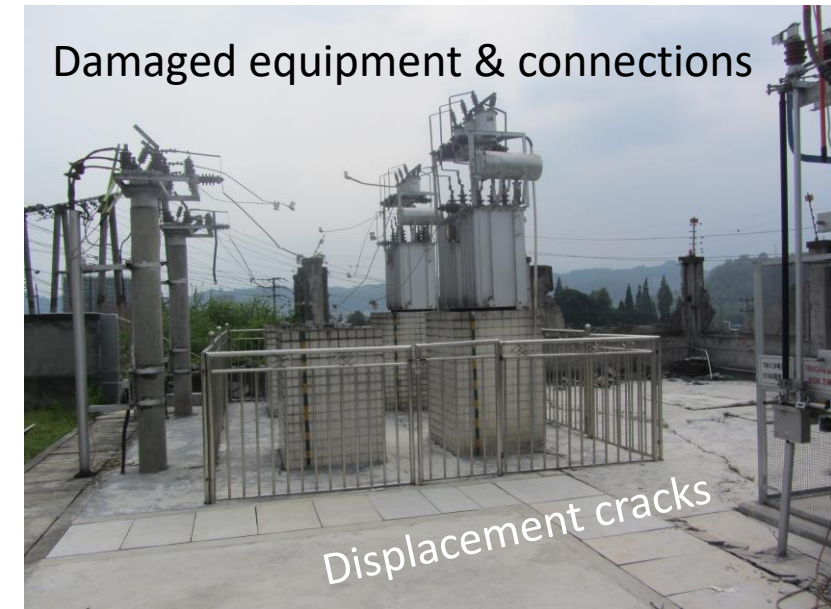
Resulted in ~3" settlement, ~6" horiz. movement
