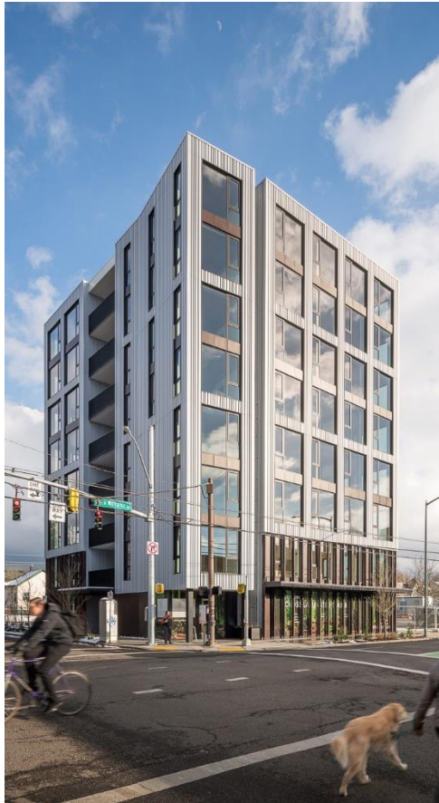
Carbon 12 Building, Portland OR
