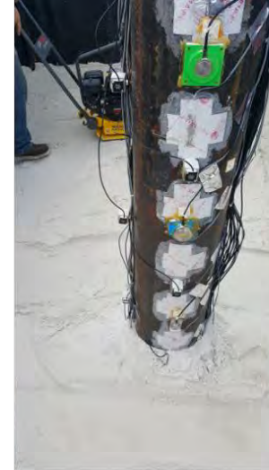
d). Compaction of dense layer
