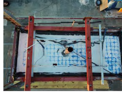
c). Drone Picture from above the box
