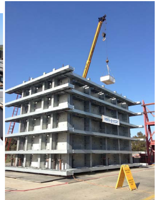
Hopper and crane method (fast and expensive)
