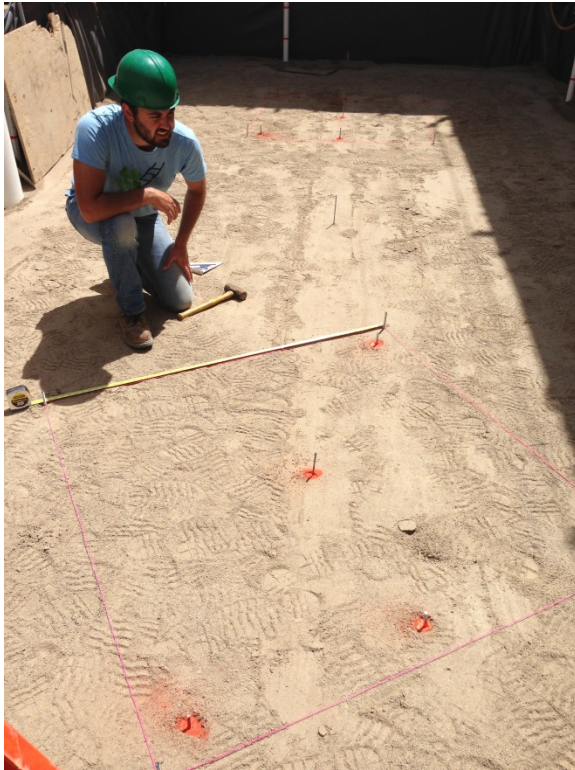
Marking of locations before placement
