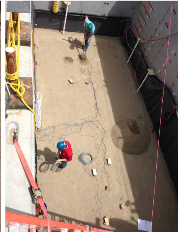
Covering with soil and cables running
