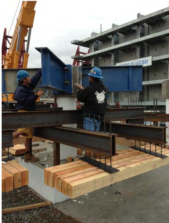
*Placement of mass support steel beams*
