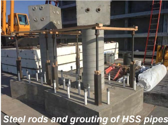
Steel rods and grouting of HSS pipes
