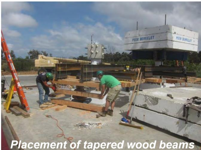
Placement of tapered wood beams
